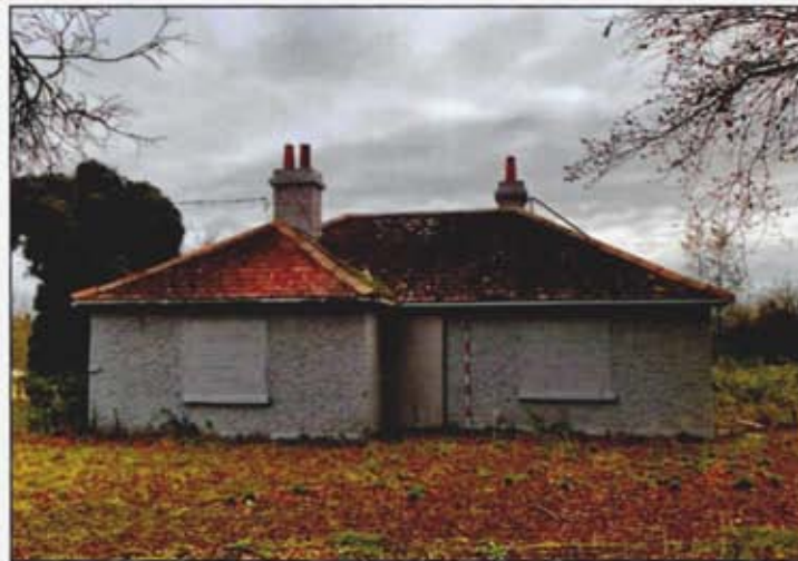
Figure 16.41: Toberbunny Lodge, north-west façade
