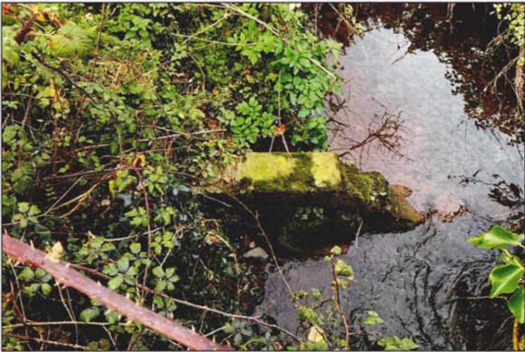
Figure 16.48: Remains of earlier bridge on west side of modern crossing
