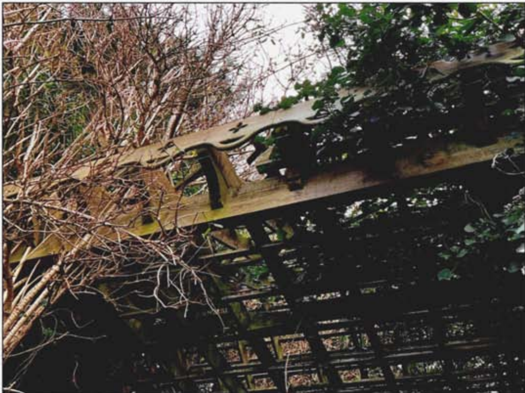
Figure 16.37 Decorative trim on new roof timbers on late 19th century house
