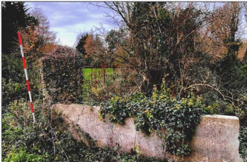
Figure 16.50: Modern bridge crossing facing south-west, showing gate pier to south
