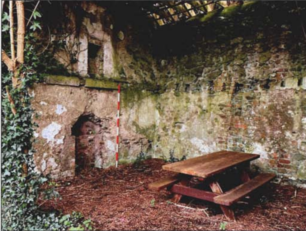
Figure 16.36 Interior of late 19th century house, showing new roof timbers, fireplaces in west gable and blocked-up doorway in north wall
