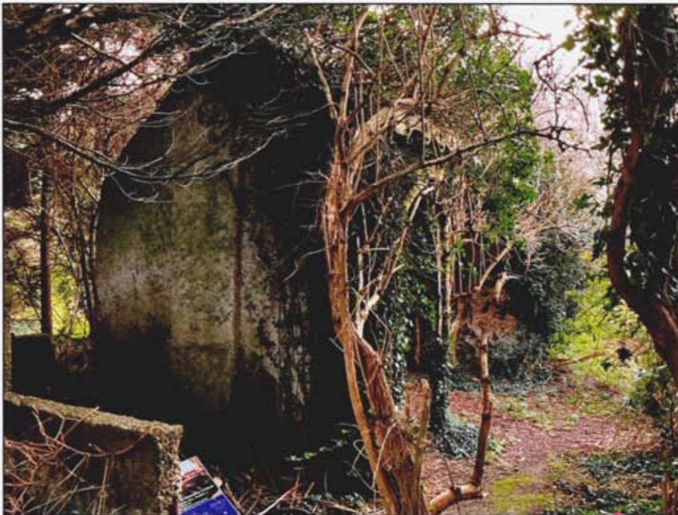
Figure 16.35 West gable of late 19th century house
